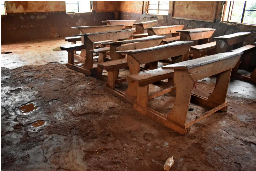
Figure 5.1. Classroom at Shimbwe Chini Primary School before renovation. Source: ↑C-re-aid (2021)
